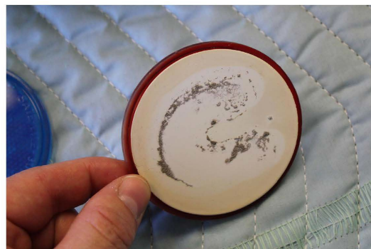
Damaged adhesive on the back of a fallen reflector.
