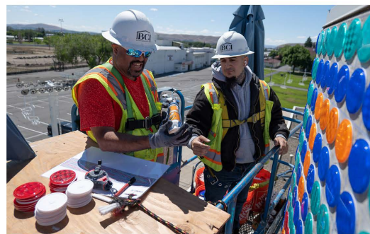
Workers with Burton Construction, Inc. apply adhesive to the back of a reflector. Photo by Yakima Valley Photography.
